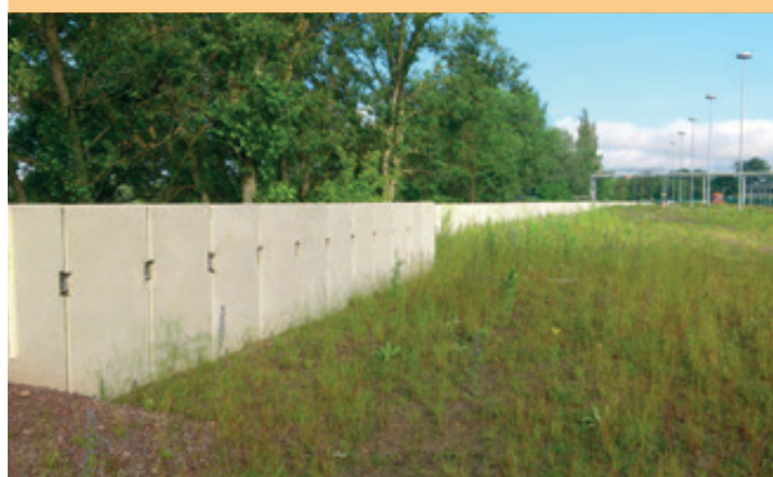
Flood protection wall, Wittenberge
