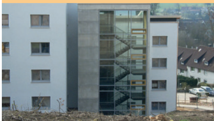
Elevator shaft with staircase, Ennepetal
